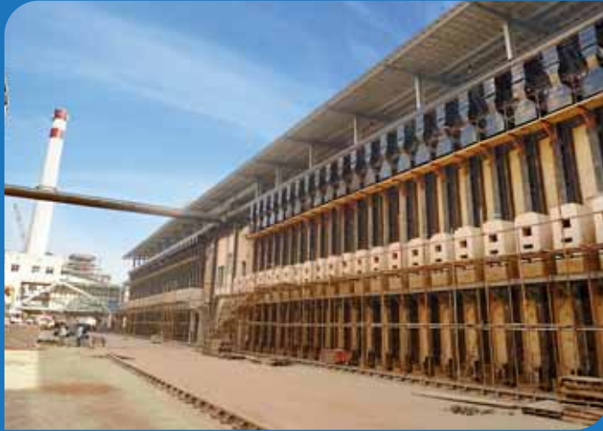
Vertical Coke Oven Battery
